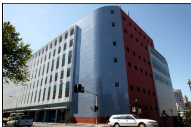
ac3's second data centre is located within Global Switch, on the outskirts of the CBD.
